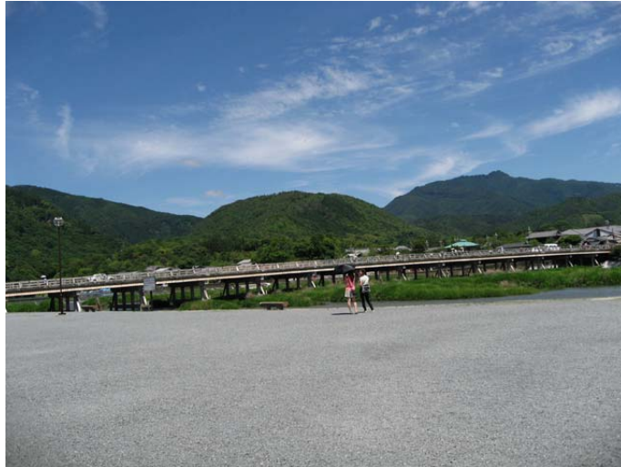
PICTURE 13 – Togetsugyou Bridge in Arashi Yama
